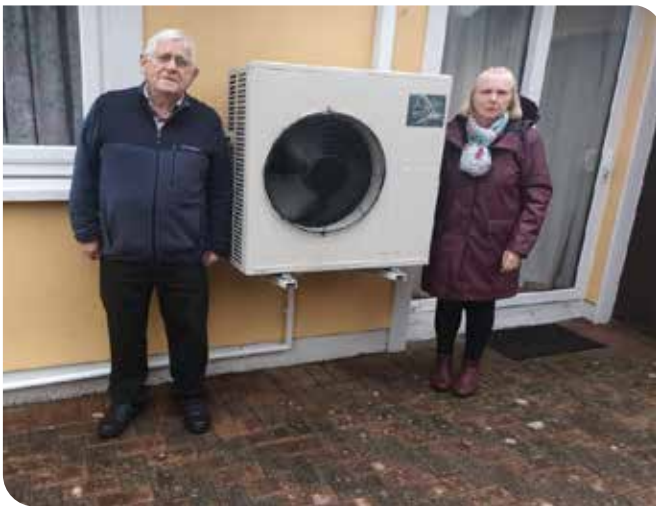
Members Pat O'Toole and Marie Ruanne of the St Patrick's Conference Westport pictured beside a newly installed heat pump.
